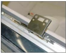
Align the edge of spacer and the rear edge of the opening of the lift wedge.
