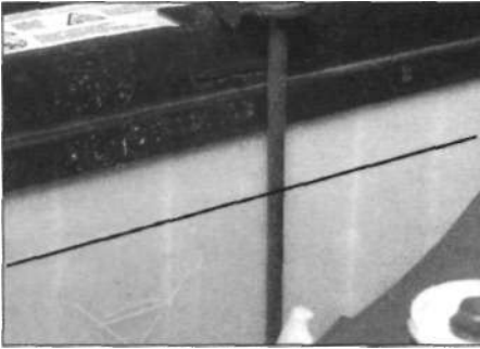
2.9a Minimum electrolyte level mark on the front of the battery
