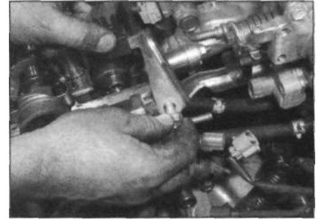
9.15 Unbolting the lifting eye and air chamber support bracket
