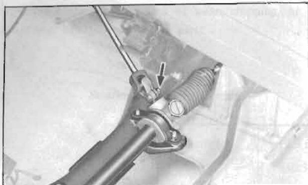
Fig. ST-13 Disconnecting lower joint from pinion
