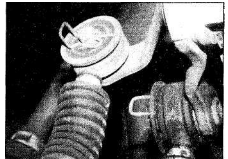
2.1 Prise out the clips and disconnect the gearchange cables from the levers
