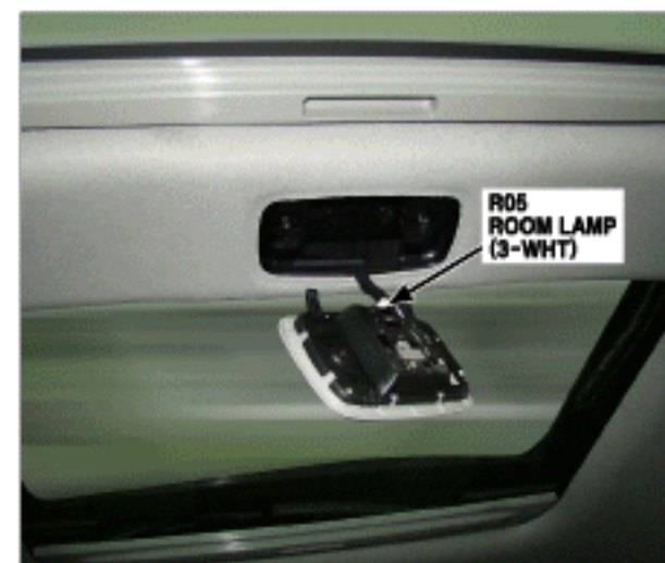
90. Center of Roof Trim
