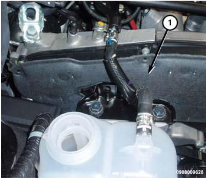
Fig. 246: Upper Timing Cover Insulator Courtesy of CHRYSLER GROUP, LLC
