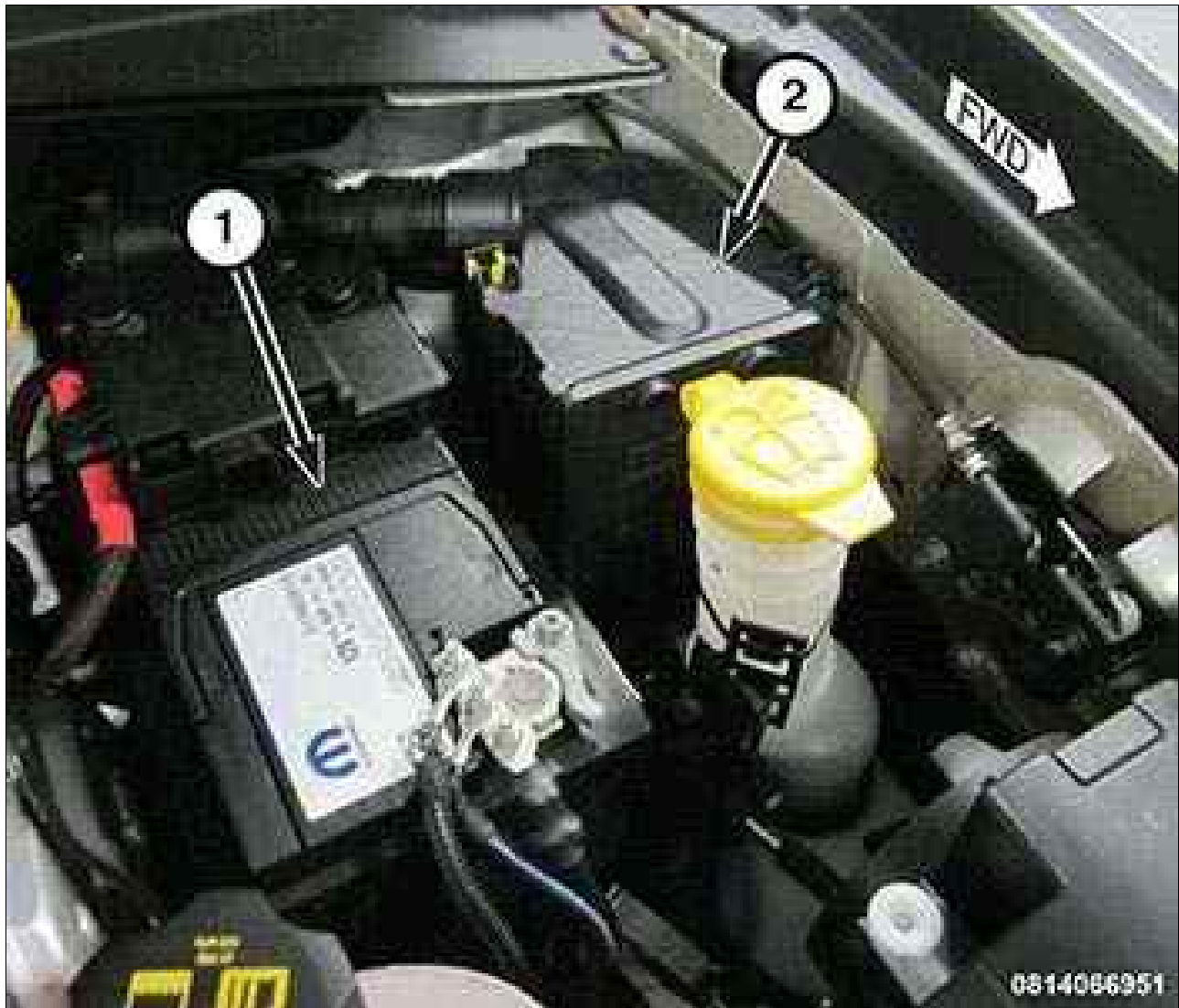
Fig 1: Battery & Power Distribution Center
