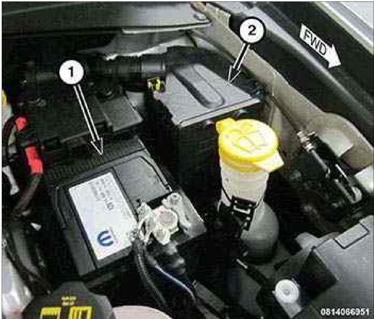
Fig 1: Battery & Power Distribution Center
