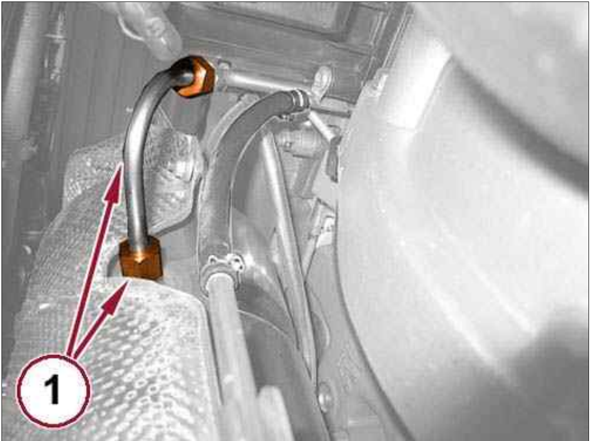
Fig 5: Upstream Pressure Sensor Pipe Fittings
