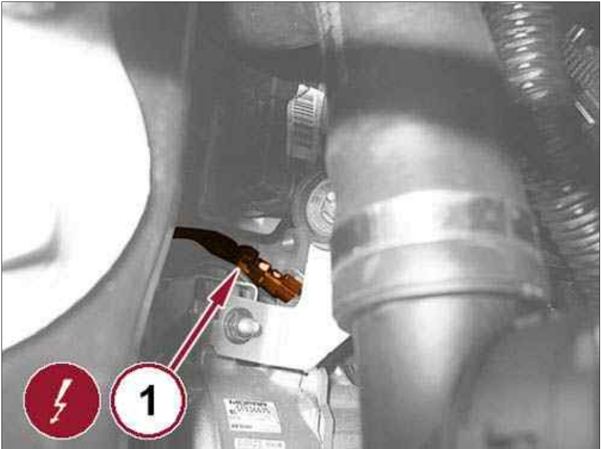
Fig 7: Upstream Exhaust Gas Temperature Sensor Electrical Connection
