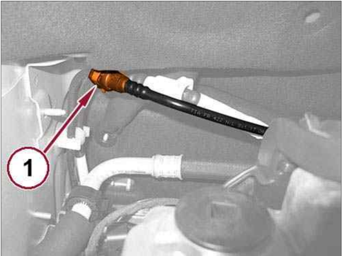
Fig 3: Front Fuel Delivery Line Right End Quick Coupling
